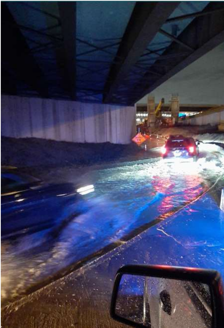
Terminal A to B – IP Southbound No SWPPP protection of inlet
