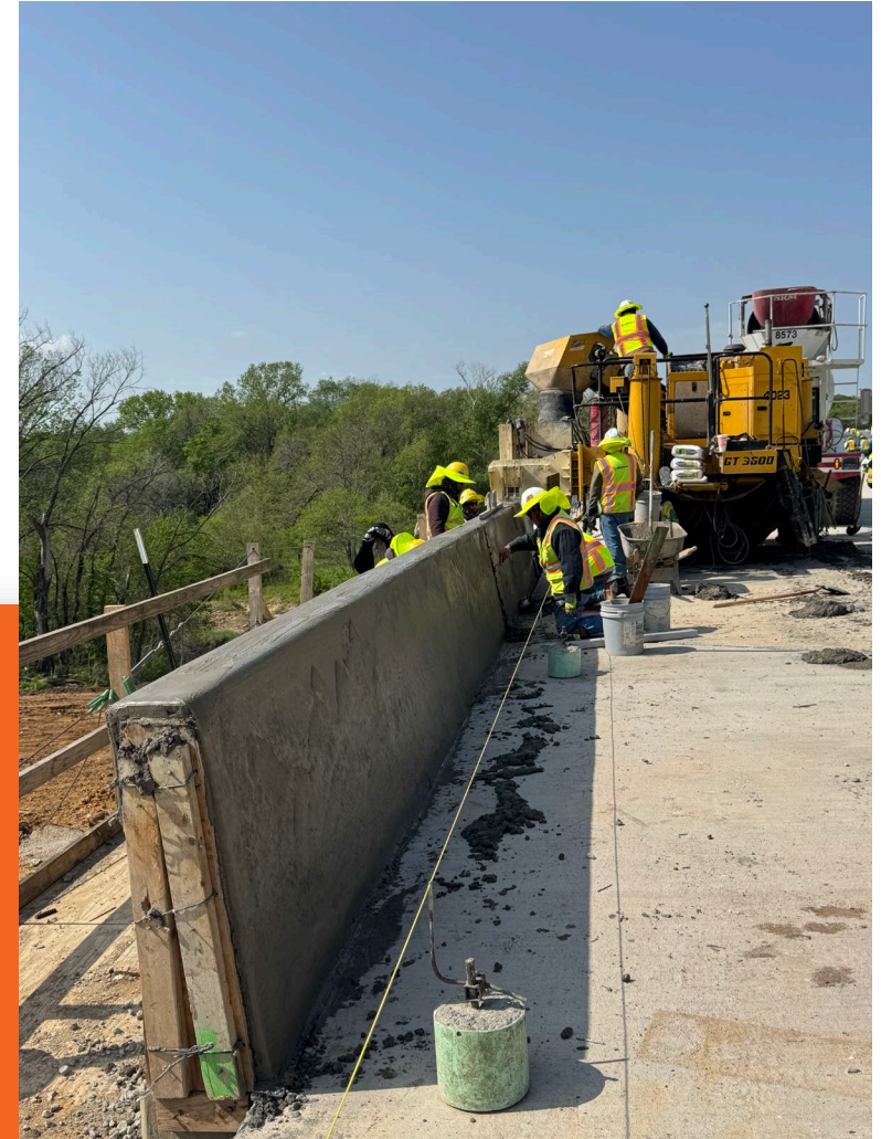
Bear Creek Bridge SSTR Concrete Rail Preparation
