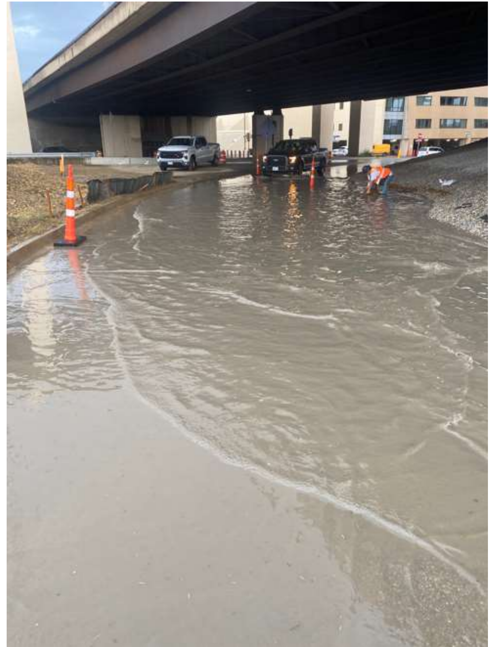
Terminal C to D – IP Southbound Swale blocking the inlet
