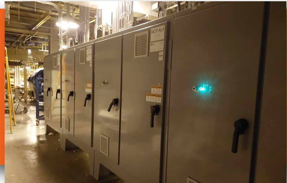
Terminal D Phase 2 – New Motor Control Panels
