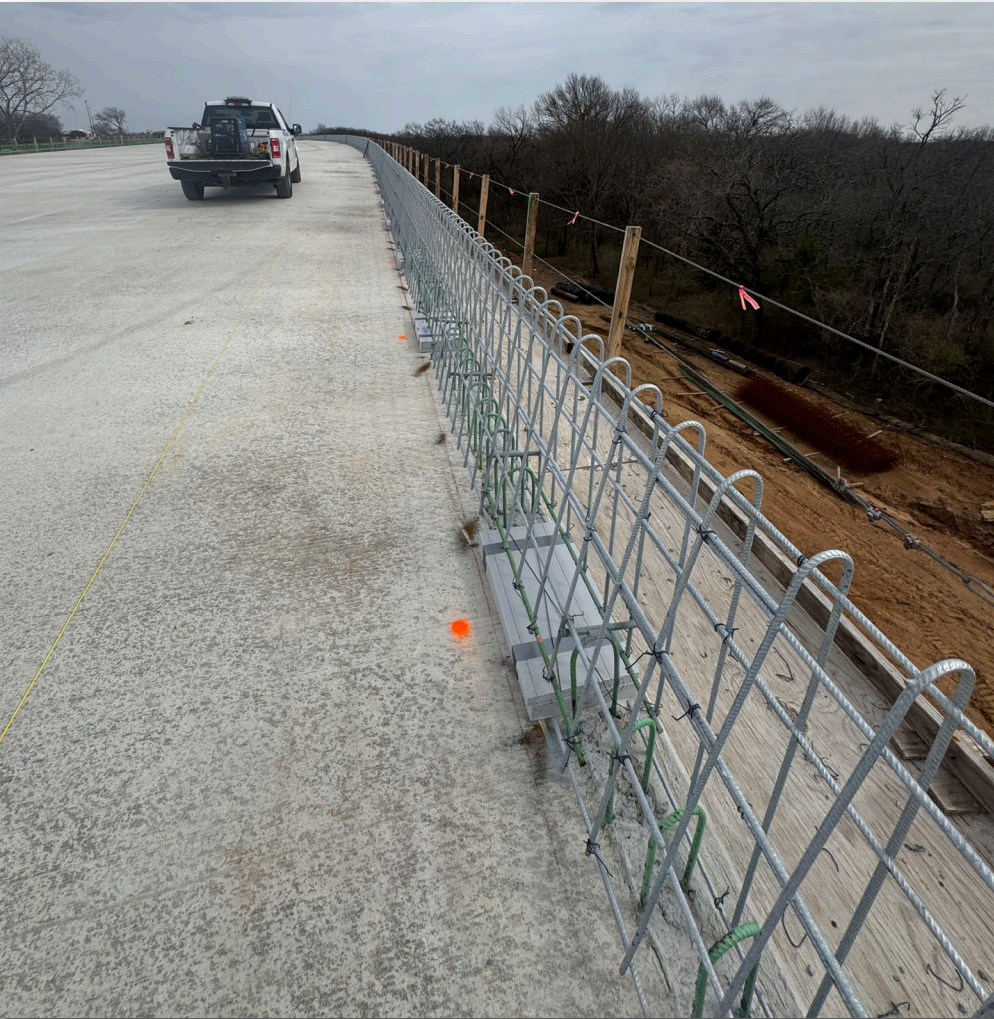
Trigg Lake Bridge Concrete Rail Preparation
