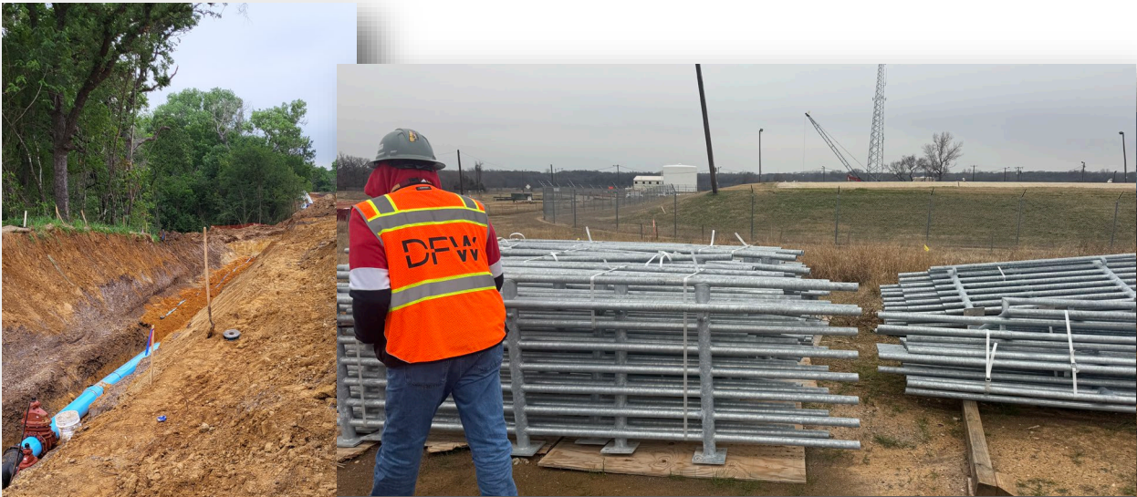
Pedestrian Rail for Emergency Spillway Stored On-Site
